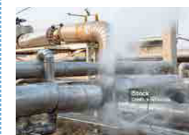
Flue Gas Desulfurization
